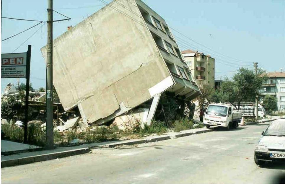
Figure 2. Failure in the form of soft storey mechanism (Kocaeli, 17 August 1999 Marmara earthquake)
